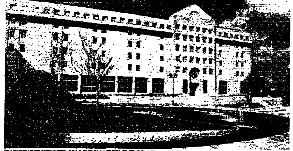
EDINBURGH SHERATON HOTEL: 7.5 MILES FROM AIRPORT, OVERLOOKS EDINBURGH CASTLE, 263 ROOMS, HEALTH CLUB
